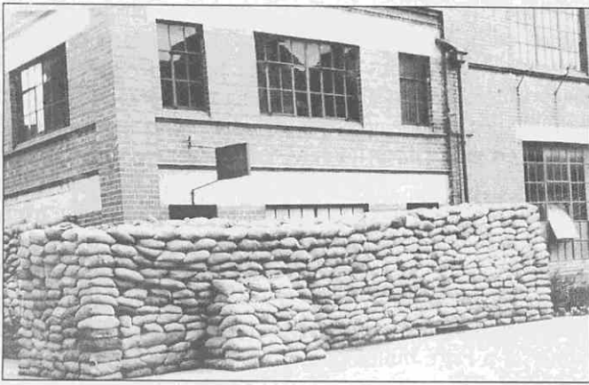
A wall of sandbags protects part of Fry's Factory against bomb blast, shrapnel and machine gun bullets in September 1939
